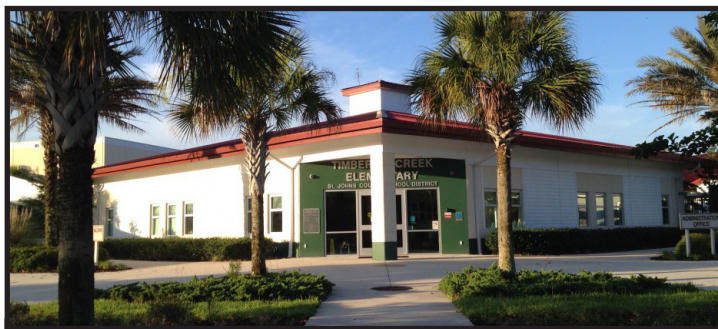
Timberlin Creek Elementary School 555 Pine Tree Lane | St. Augustine, FL 32092
