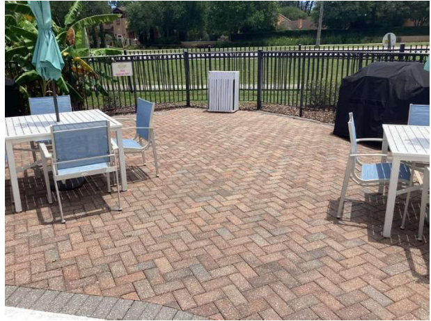
Masonry pavers overview
