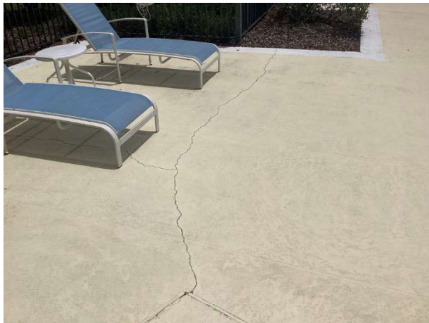
Concrete cracks
