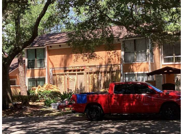
Current stucco repairs
