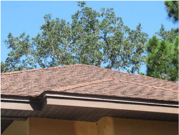
Beachside clubhouse roof
