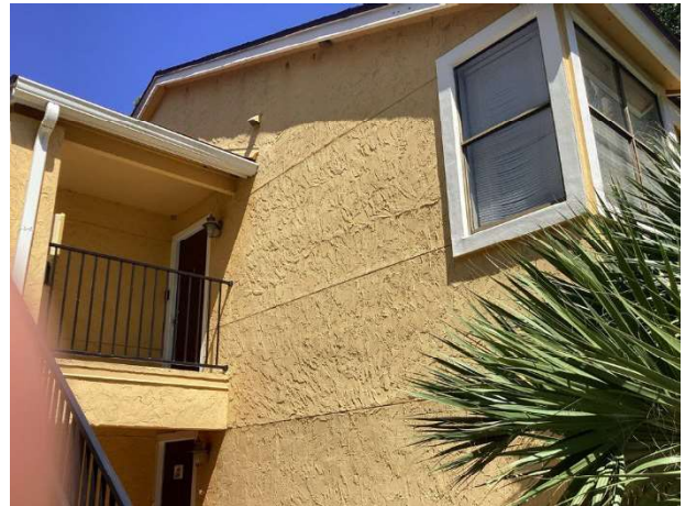
Stucco wall finishes
