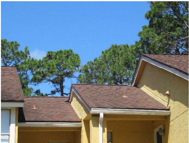
Beachside asphalt shingle roofs
