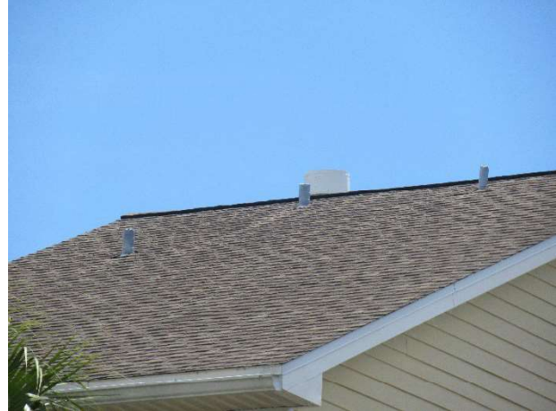
Golfside asphalt shingle roofs
