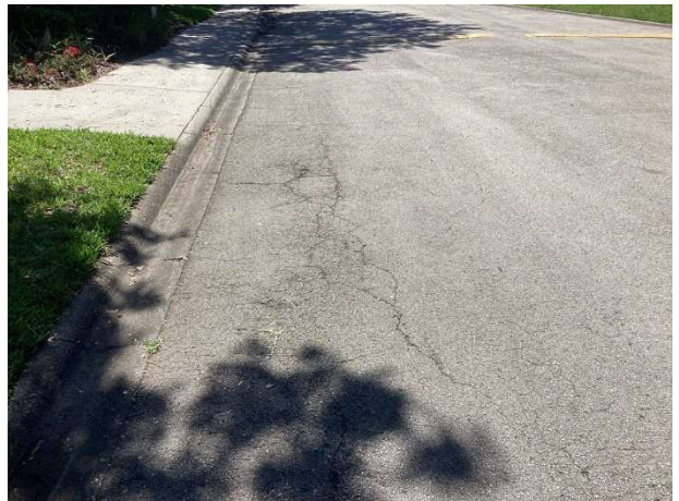
Pavement cracks
