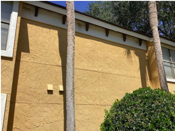
Stucco wall finishes
