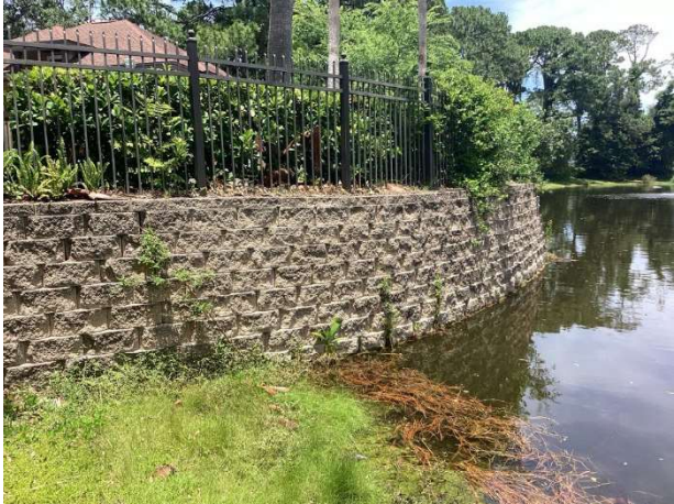
Masonry retaining wall
