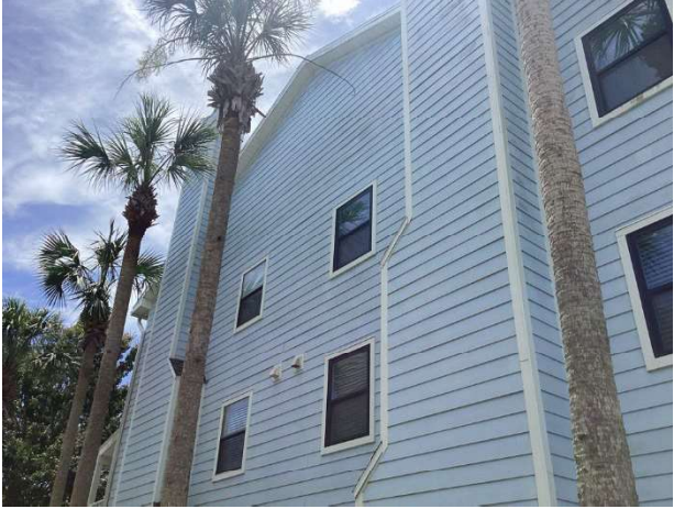
Fiber cement siding
