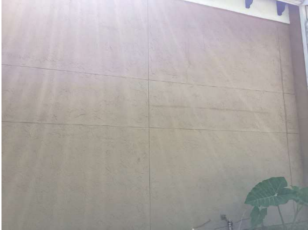
Stucco wall finishes
