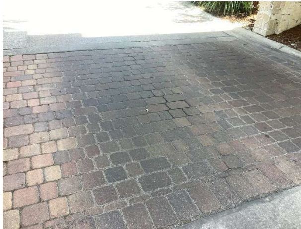
Masonry pavers overview
