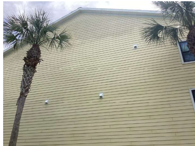
Fiber cement siding
