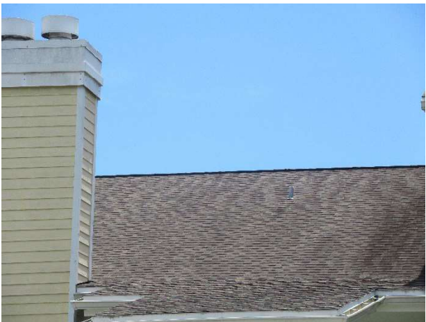
Weathered shingles at Golfside buildings
