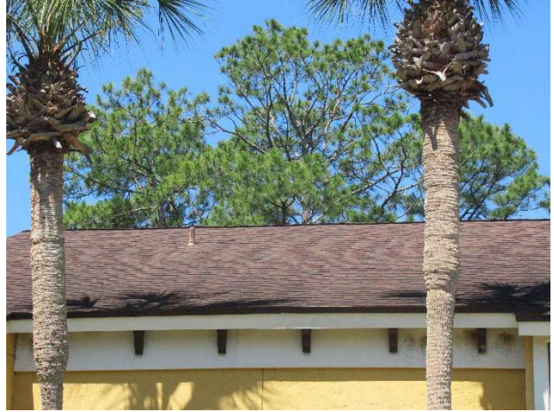
Beachside asphalt shingle roofs
