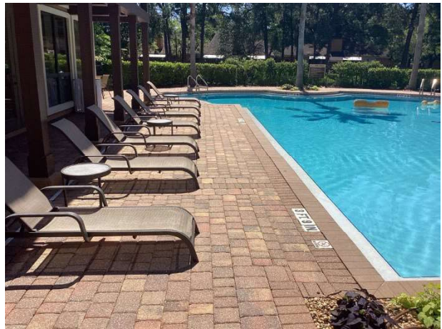
Paver pool deck overview
