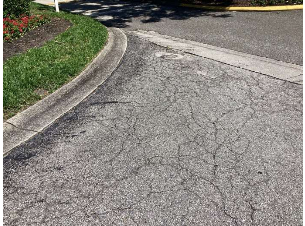
Pavement cracks
