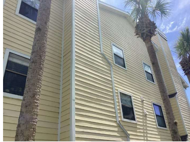
Fiber cement siding
