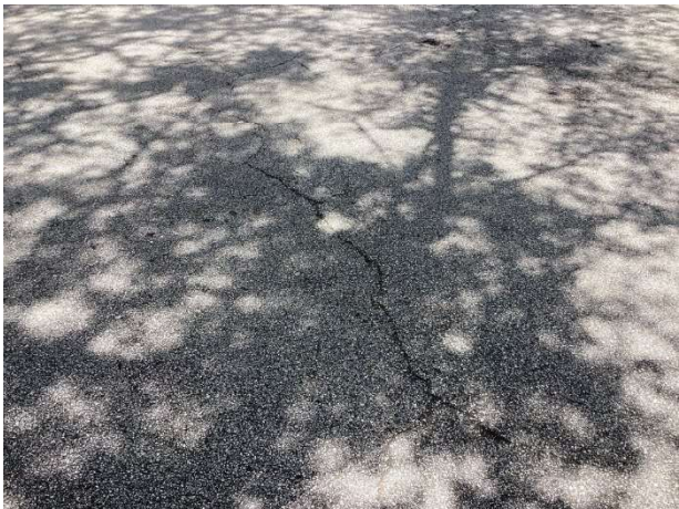
Pavement cracks
