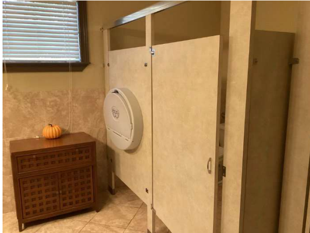
Clubhouse rest room
