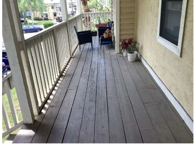
Original breezeway overview
