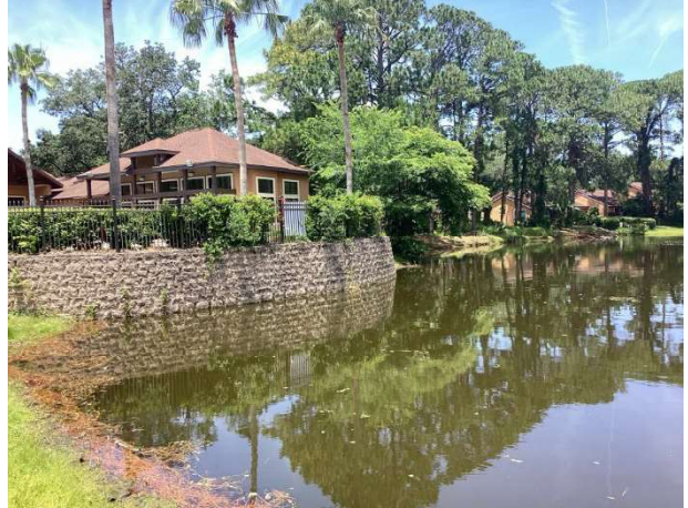
Masonry retaining wall
