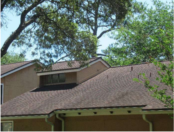
Beachside asphalt shingle roofs
