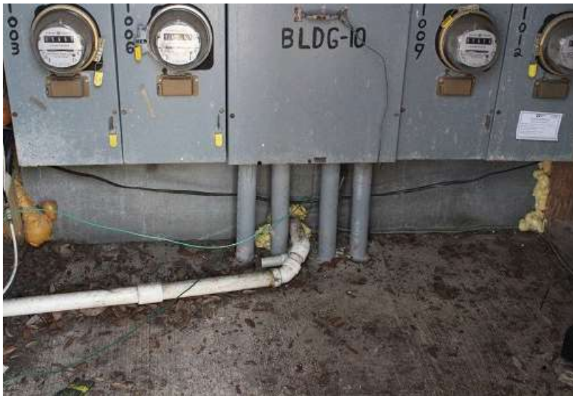
Typical foundation with no cracks
