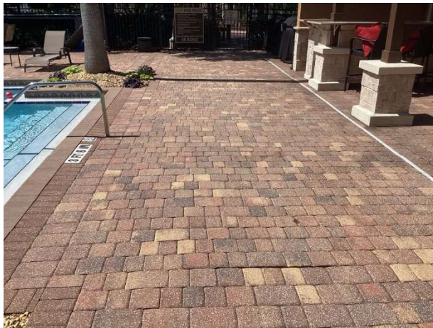
Paver pool deck overview
