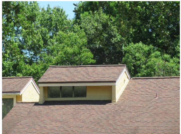
Beachside asphalt shingle roofs
