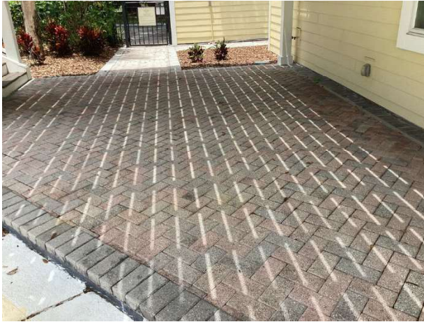
Masonry pavers overview
