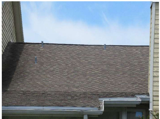
Golfside asphalt shingle roofs
