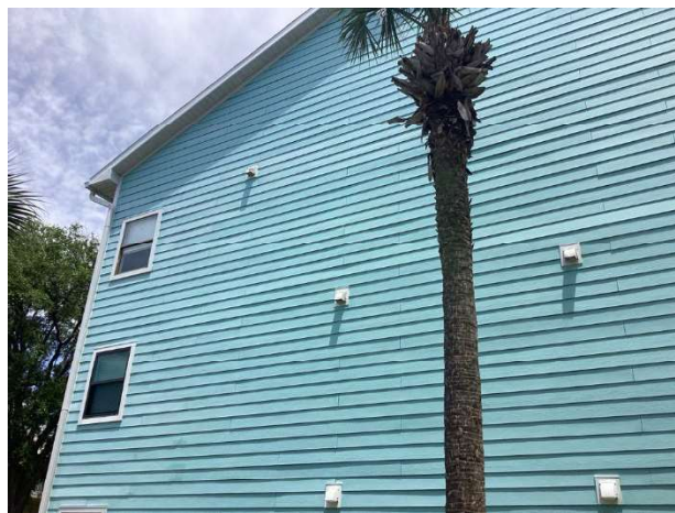
Fiber cement siding
