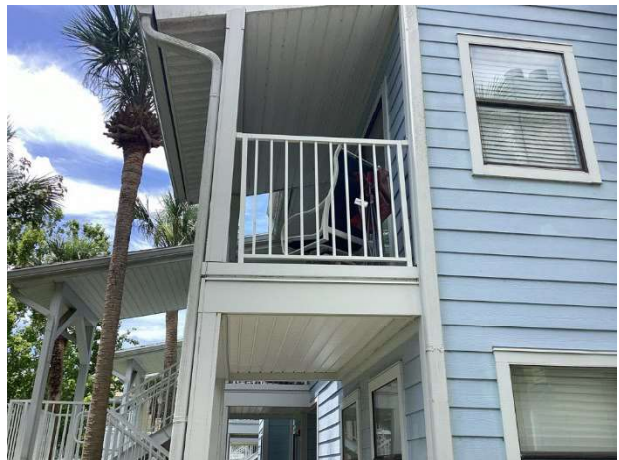
New balcony overview
