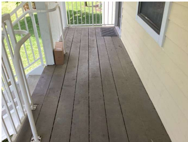
New balcony overview
