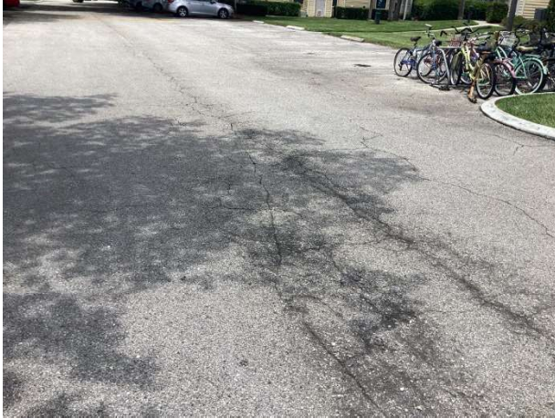
Pavement cracks
