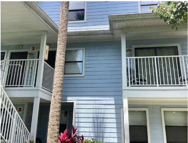
Fiber cement siding
