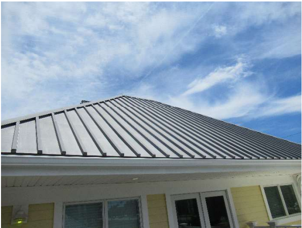
Metal roof at Golfside clubhouse
