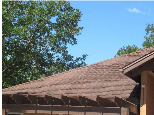
Beachside clubhouse roof
