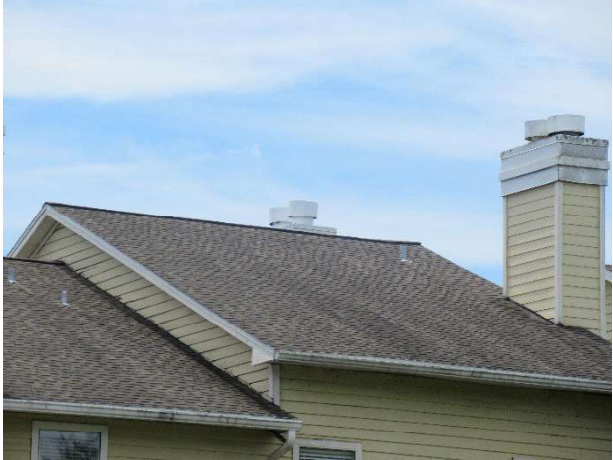
Weathered shingles at Golfside buildings
