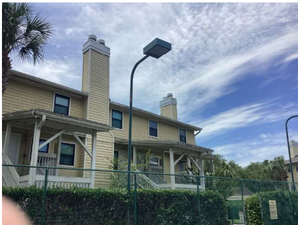
Light pole and fixture
