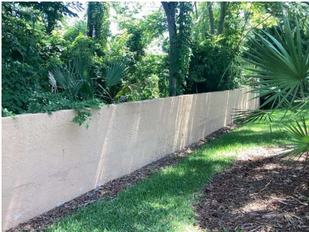
Stucco perimeter wall overview
