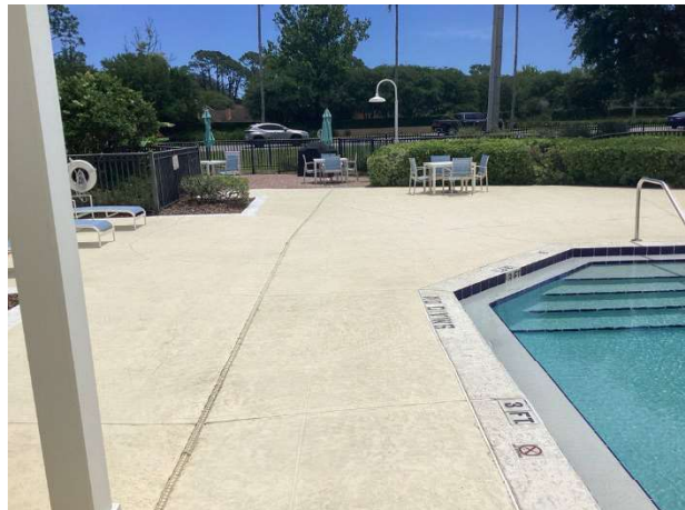
Golfside concrete pool deck
