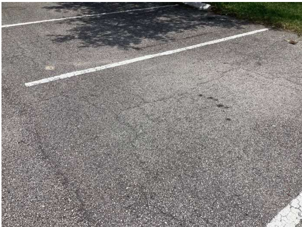
Pavement cracks
