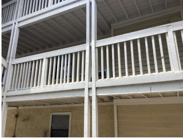
Original breezeway overview
